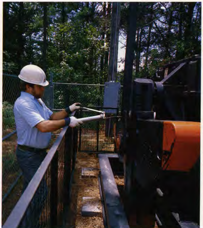
Structural bearings can be easily lubricated from the ground.
