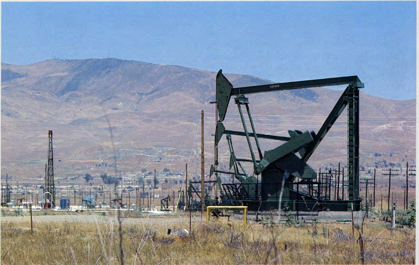
LUFKIN M-228D-173-100 Units, Chevron USA, Fresno County, California.
