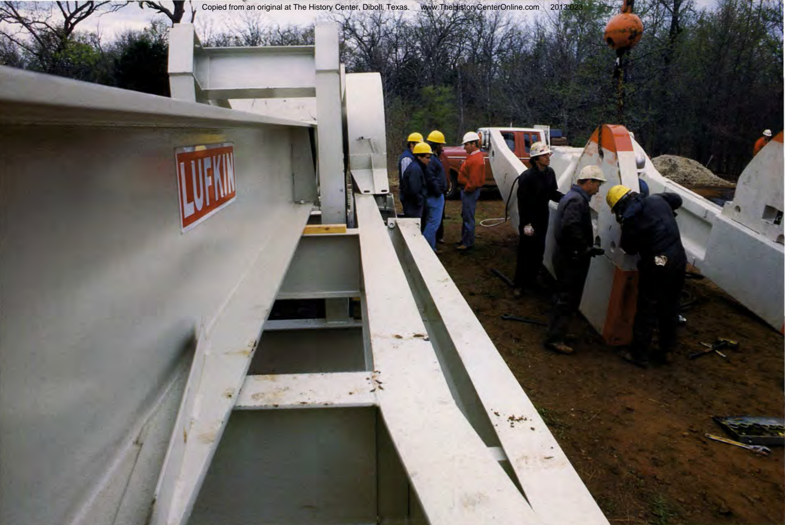
(Above) Handling the 18-ton gear reducer and cranks for a M-912 unit requires special rigging by the installation crew, especially during the assembly process when the massive and awkward piece must be lifted relatively level. (Left) LUFKIN sales and service representative Rick Hughes (red jacket) visits with employees from the plant, (l-r) Vernon Speicher, Jr. engineering oil field design group; David Jenkins, machine shop; Mike Whitten, machine shop, and Jeff Lankford, foundry engineering.
