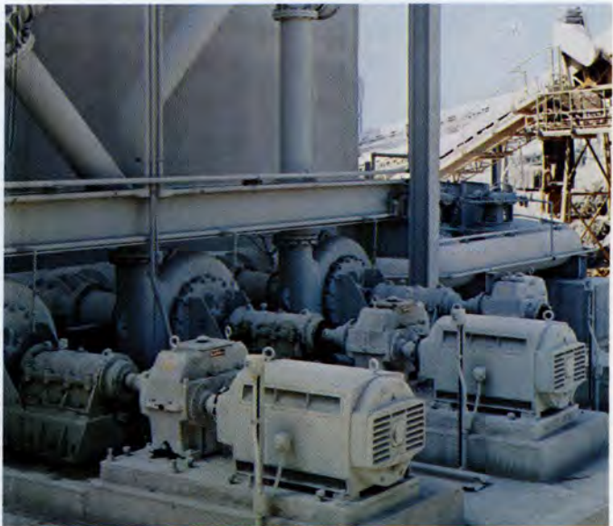
THREE of five LUFKIN S-127C reducers drive slurry pumps. TXI and subsidiaries make a variety of concrete products
