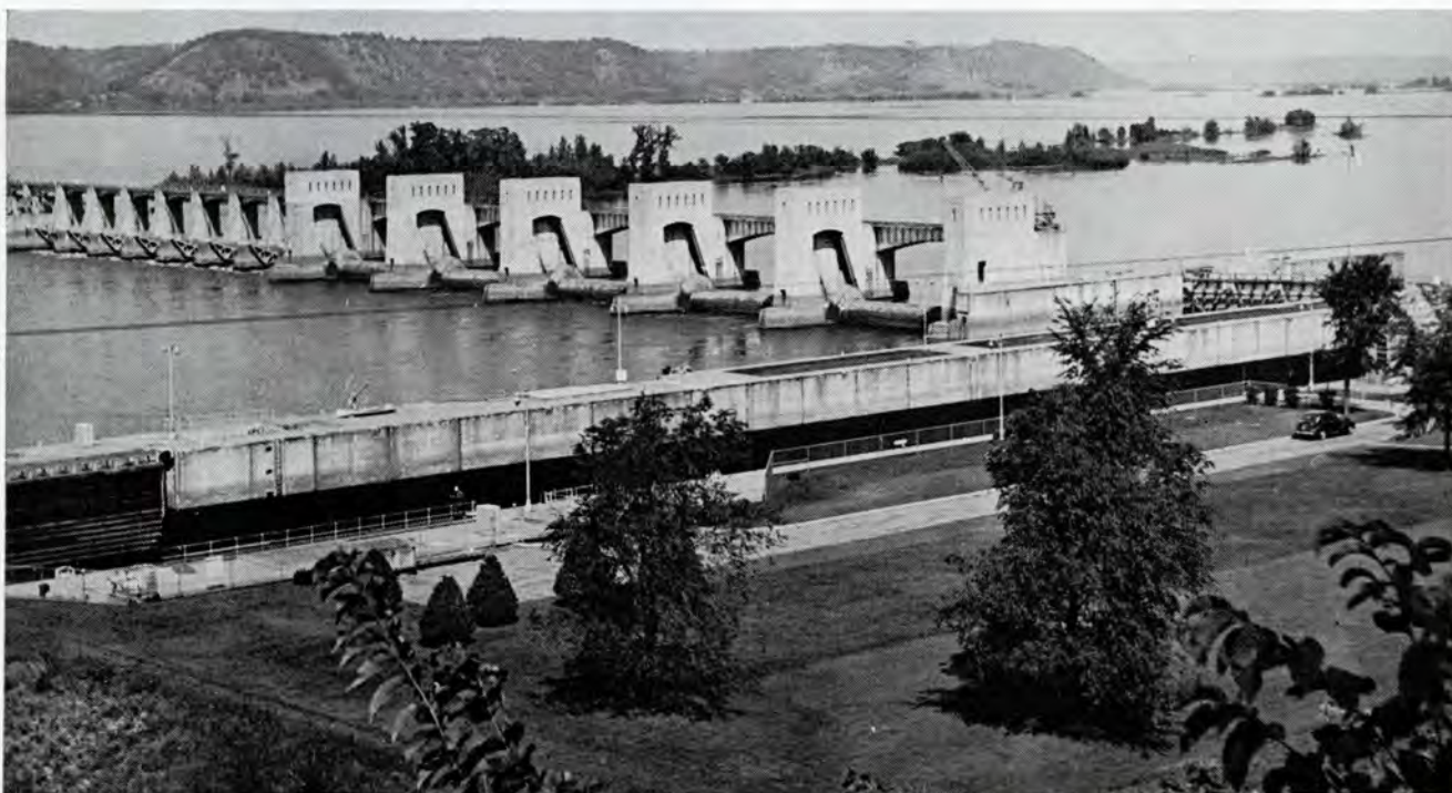
AT LYNXVILLE, a multi-million dollar dam and lock make possible 651 miles of river navigable
