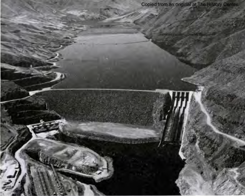
THIS is Brownlee Dam, first unit of Idaho Power Company's new three-dam development in Hells Canyon between Idaho (left) and Oregon. At right is the spillway which is as tall as a 14-story building. About a mile upstream is fish facility used to collect ocean-bound salmon for hauling in custom-built trucks around the dam
