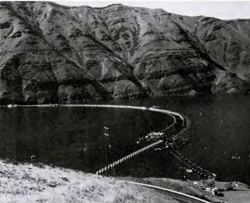
OVER-ALL view shows downstream-migrant fish facility, first of its kind ever built, that Idaho Power Company operates in the Brownlee reservoir to give safe passage to ocean-bound salmon and steelhead fingerlings
