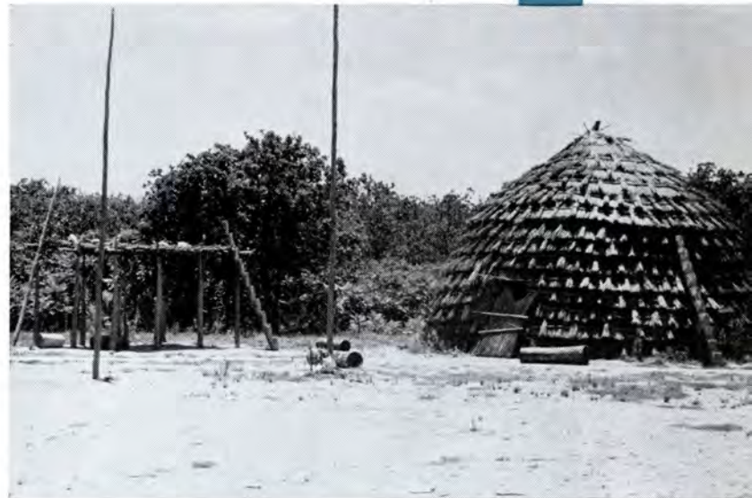
THIS is a Wichita grass house with a work arbor on the left. Notched pole leaning against work arbor and grass house were used by Indians as a ladder
