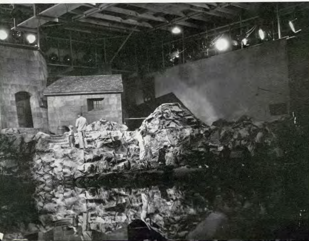
MAINE COAST IN HOLLYWOOD. At the base of the lighthouse set on the huge, new Will Rogers Memorial Stage. The tank is 80 ft. square, contained more than 100,000 gallons of water, and the set weighs considerably more than 1,000,000 pounds.
