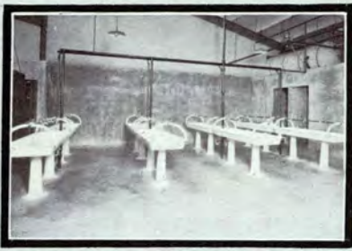
MODERN SANITARY WASH ROOMS FOR EMPLOYEES
