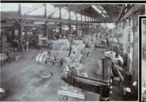
GENERAL VIEW OF MACHINE SHOP LOOKING NORTH
