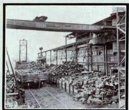
FOUNDRY YARD SHOWING TRAVELING CRANE WITH ELECTRIC MAGNET
