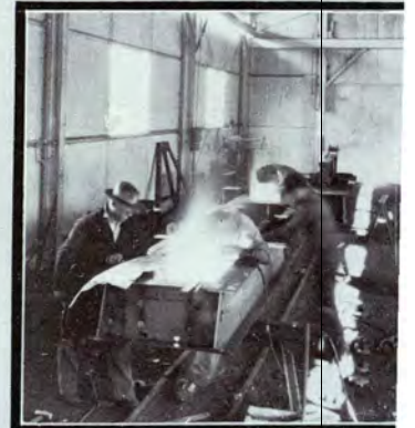
ARC WELDING OF BED PLATE
