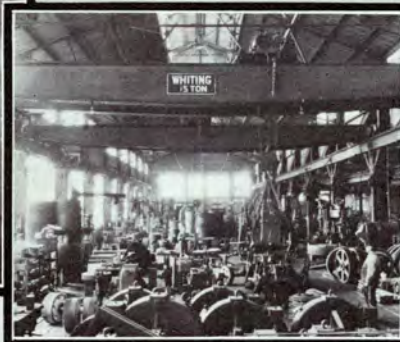
SECTION OF MACHINE SHOP NOTE ELECTRIC CRANES
