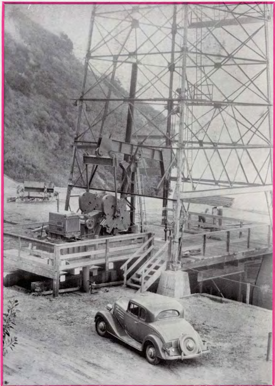
At left—Atlantic Oil Producing Company, Gates Lease, Great Bend, Kansas, Lufkin No. TC 3-18 Unit and auxiliary equipment.
