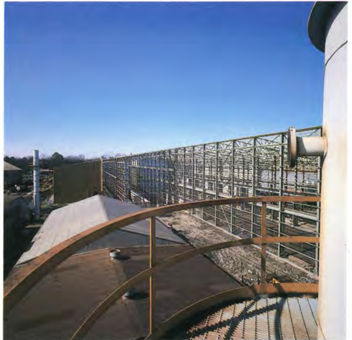
Completion of a new large castings foundry has been delayed
